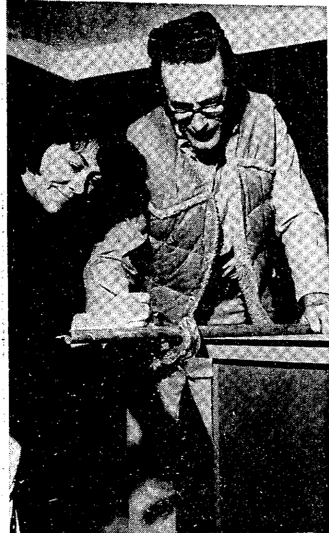
CRISIS CENTER — Cleone Smith, chairman of the new Crisis Assistance Center at 2504 Adams, helps workman Russell Speirs finish off plumbing improvements at the new facility for retarded persons.
